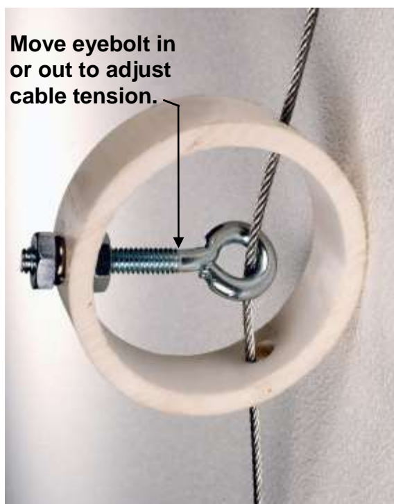
Photo # 5.31 (Cable Adjuster Assembly)
